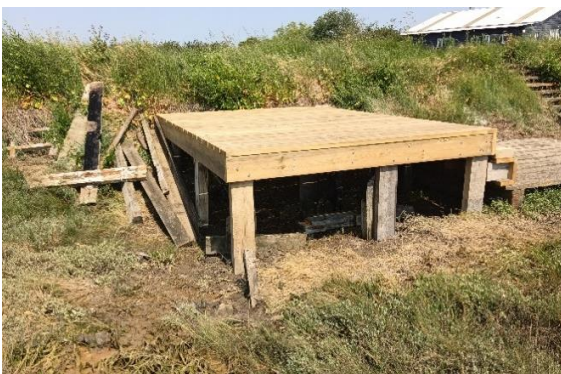
New staging for PVT jetty
